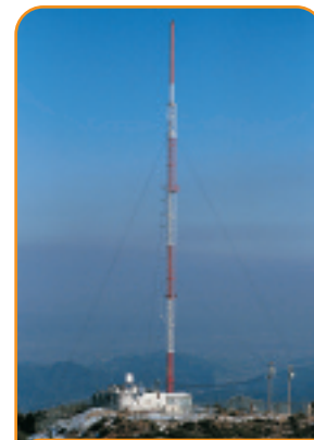
TRASAR® V-Series antenna KNTV for a channel 11 features pressurizable radome to withstand salt air coastal environment.
